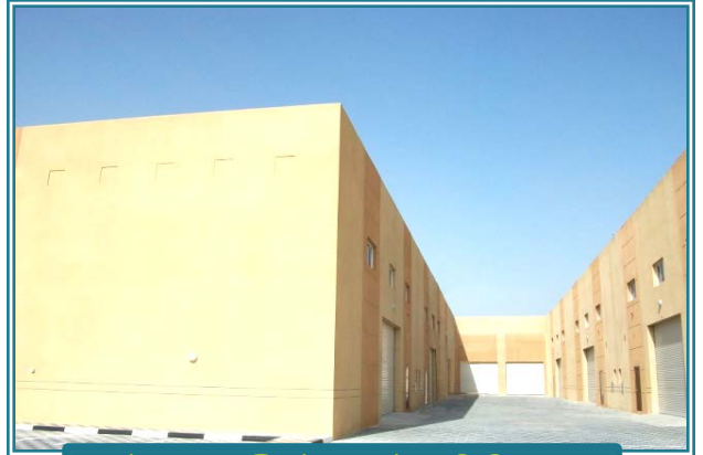
AHMED AL RAHOOMI WAREHOUSE
