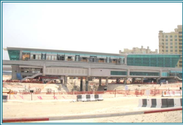
TRUMP TOWER STATION @ PALM JUMEIRAH MONORAIL TRANSIT PROJECT
