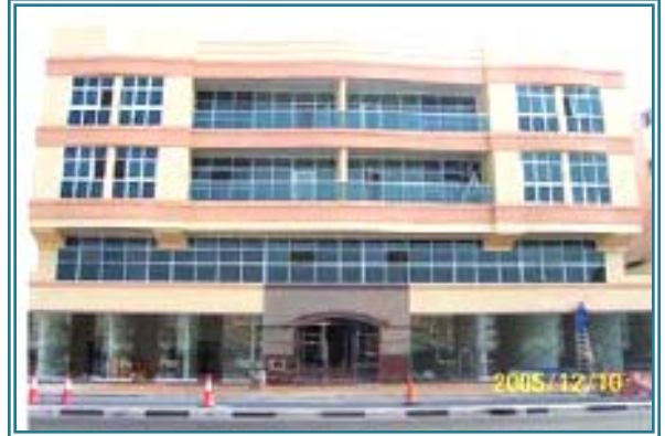
AL MANSAR COMMERCIAL BLDG
