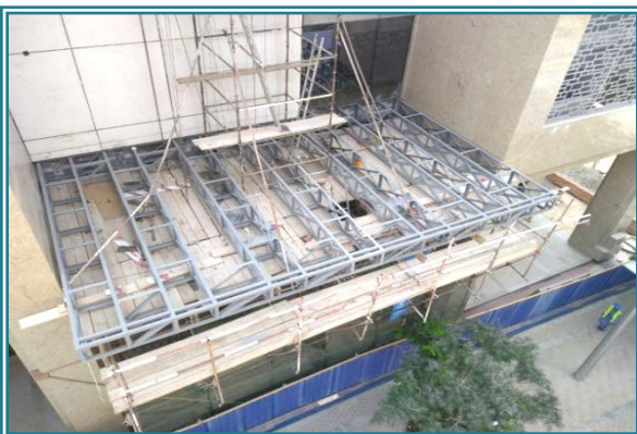
BAHWAN TOWER CANOPY
