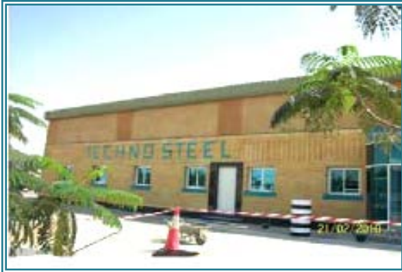
TECHNO STEEL FACTORY
