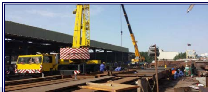
MOBILE CRANE, FORKLIFTS
