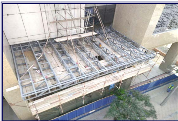
BAHWAN TOWER CANOPY
