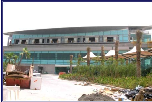
ATLANTIS STATION @ PALM JUMEIRAH MONORAIL TRANSIT PROJECT
