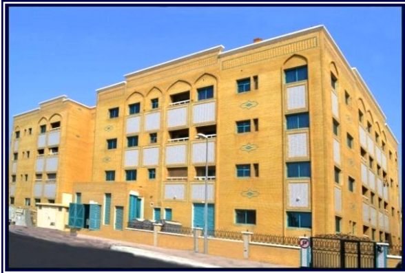
RED CRESCENT SOCIETY BLDG
