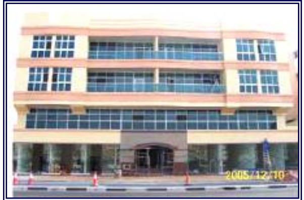
AL MANSAR COMMERCIAL BLDG
