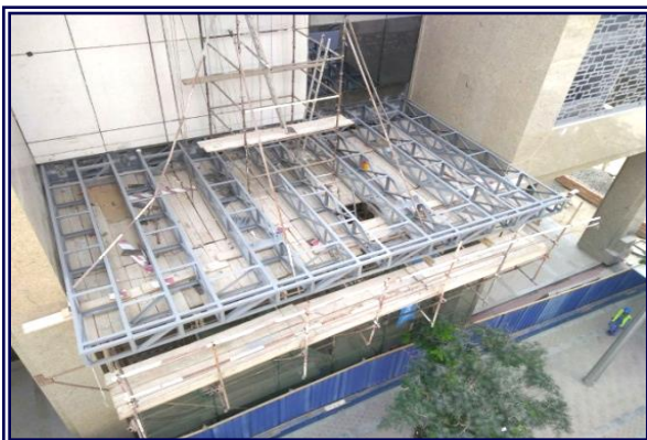
BAHWAN TOWER CANOPY
