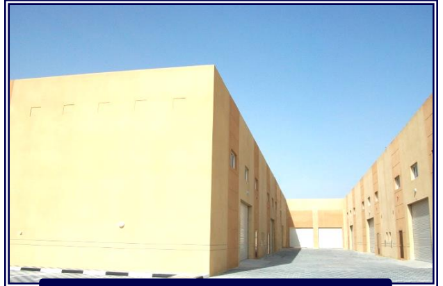
AHMED AL RAHOOMI WAREHOUSE
