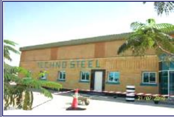
TECHNO STEEL FACTORY
